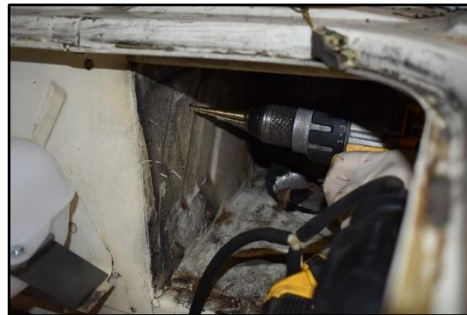
Figure 11-8: Drilling holes for plate mounting.
