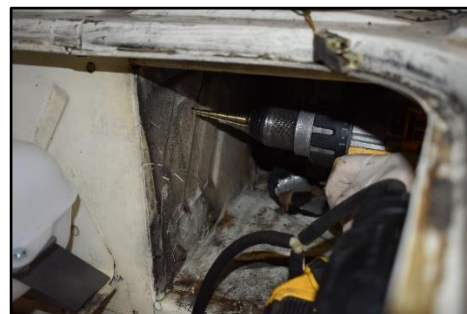
Figure 33: Drilling holes for plate mounting.
