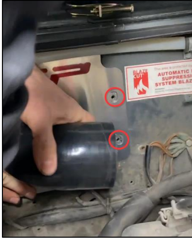
Figure 58: Air intake panel installation.
