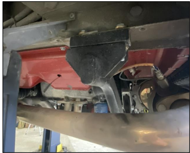
Figure 6: 2WD Vanagon rear crossbar install with spacers.
